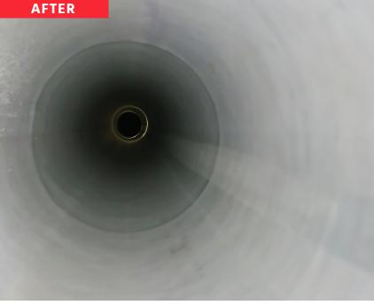
PTI Pressure is an approved installer of RS BlueLine® from HammerHead® Trenchless. RS BlueLine is a cured-in-place pipe (CIPP) system for the trenchless renovation of potable water mains and other water pressure systems.
